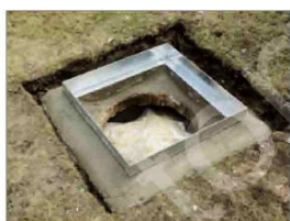
Install cover and put cement morder around
